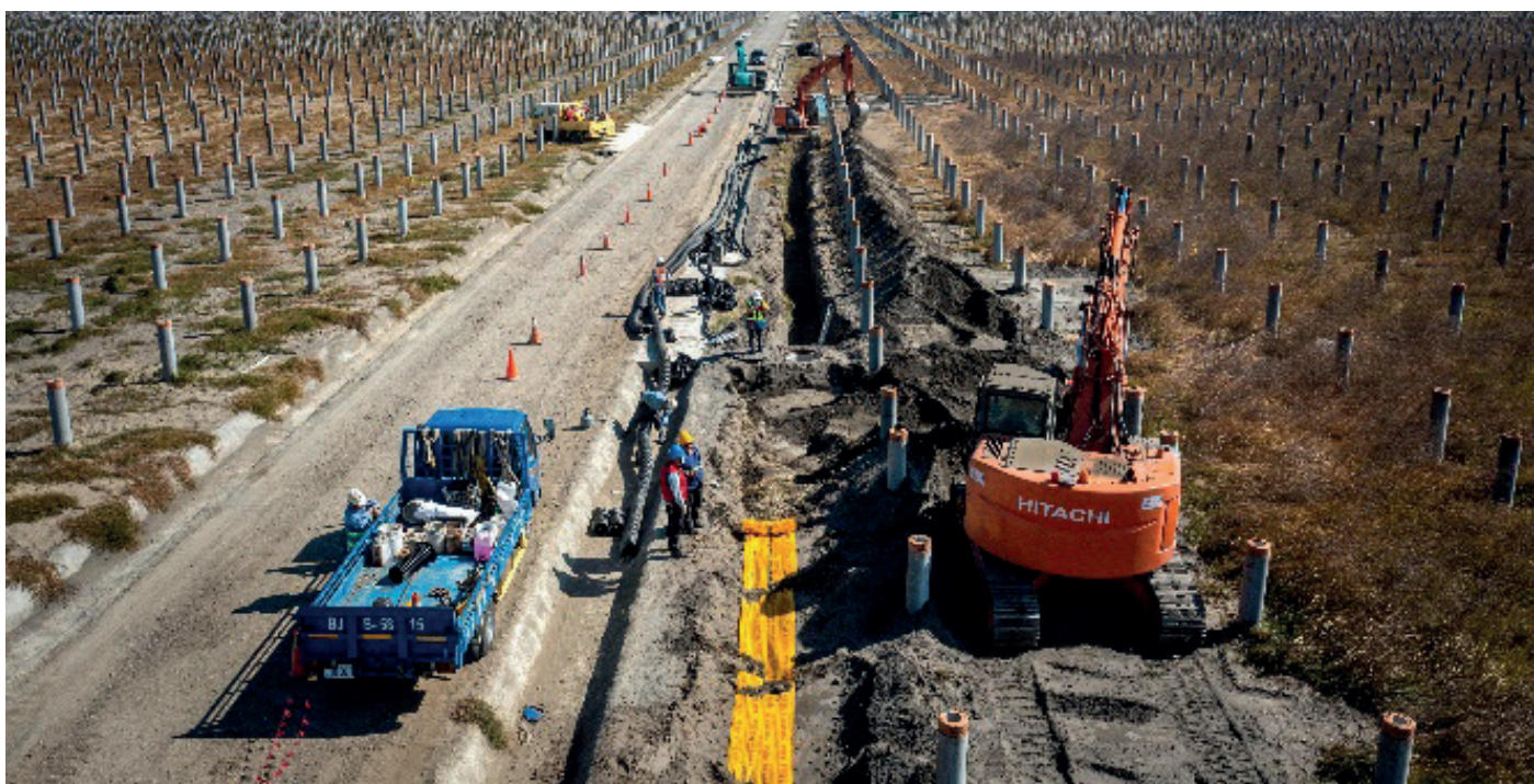
Construction of drainage canal
