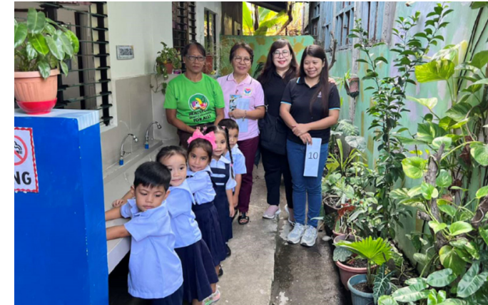
Vena Energy at a children development centre with the newly constructed Water, Sanitation, and Hygiene facilities
