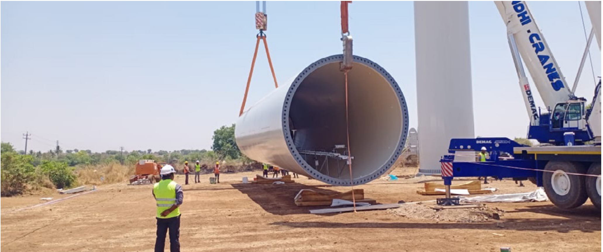
Construction site of 181 MW solar-wind hybrid project, Guddalur, India
