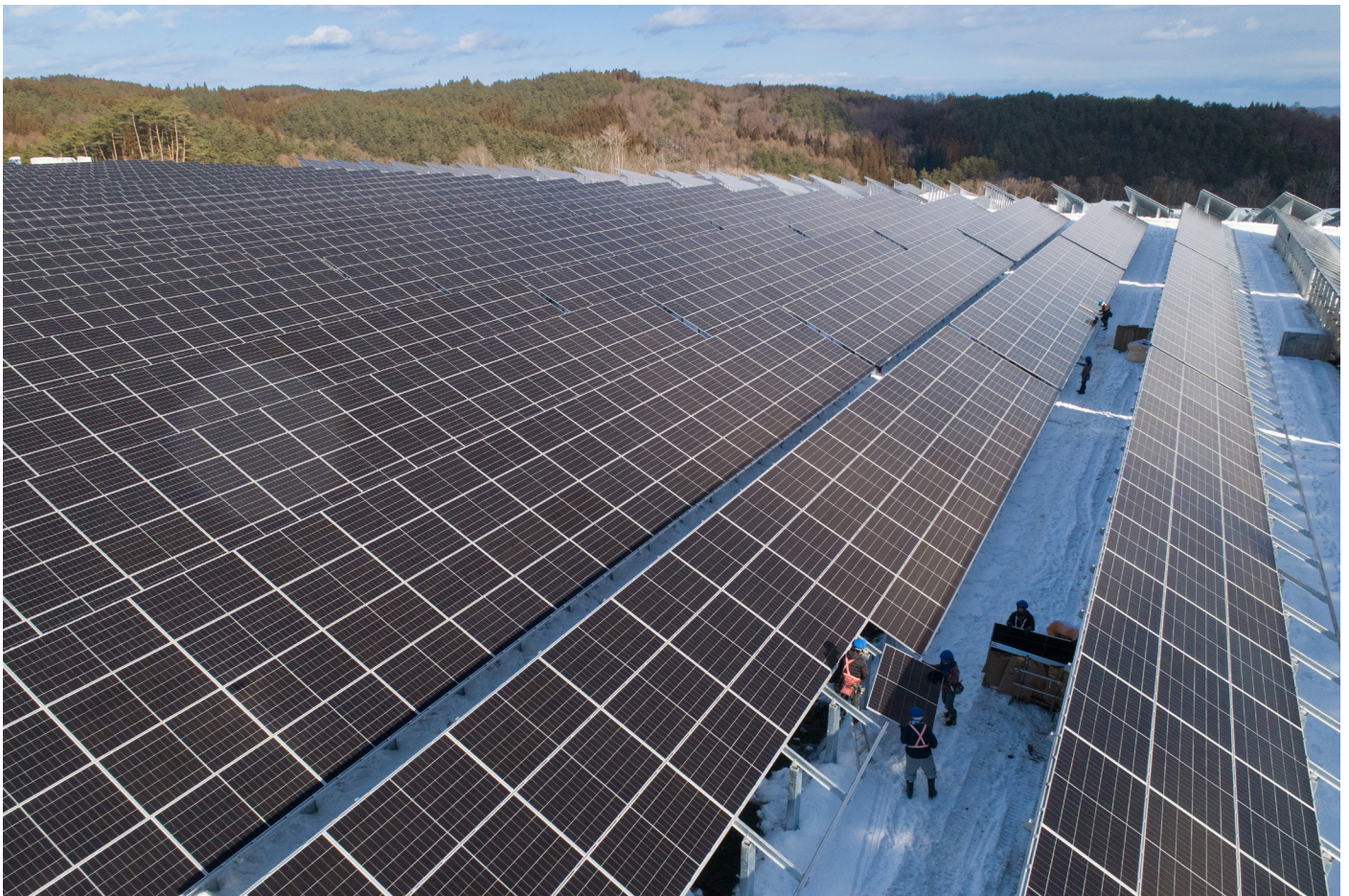
Installation of solar PV panels in Japan
